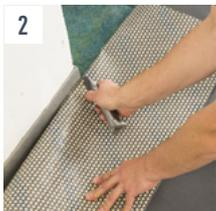
**2** Keep a distance of at least 3 mm to rising structures, for example, walls or door frames. Cut the head and edge areas exactly with the hooked blade.
