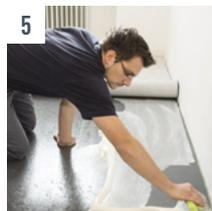
**5** Uniformly apply the UZIN dispersion-based adhesive using a notch size adapted to the structure of the back of the covering. UZIN KE 2000 S (note longer open time) is especially suitable for dense floor covering such as PVC sheets. Proceed identically with the second half of the top covering.
