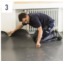
**3** Longitudinal seams between the sheets do not need to be cut. A strip of paper can be installed under the joints to prevent the underlay sheet to get stopped by the substrate.
