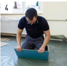
**4** Start the installation of the first row with a support panel shortened to 90 cm. To shorten the support panel, scribe the top side with a half moon blade and break off toward the top along the cutting edge. Next, cut through the XPS foam with a second cut.
