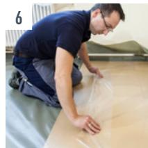
**6** Start the second row with a 30 cm long support panel and continue with full support panels. Install the panels tightly together; only production edges should form a butt-joint. Keep an adequate distance (approx. 10 mm) to the wall. Start with the installation of the top panels after the installation of the first two rows of support panels. Remove the protective adhesive film from the support panel for this purpose.
