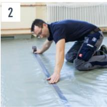
**2** Line the area to be installed in tub-fashion with a sheet of 200 µm PE film. The seam areas must overlap by approx. 20 cm. Now bond the film in the seam area with an adhesive aluminium tape over the full length.
