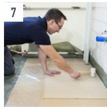
**7** Install the top panels offset to the support panel; the first row begins with a full panel and the second row with half a panel. All joints of the support panel are covered by this offset, which produces the extraordinary stability of UZIN RenoTop PLUS. Insert the top panels into the adhesive layer of the support panel and tap down over the whole surface with a rubber mallet. Make sure the abutting edges are worked exactly and tightly together.
