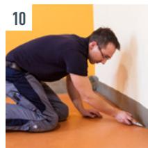
**10** The new floor covering must be installed within 48 hours after installing UZIN RenoTop PLUS. Make sure that the floor covering closes flush with the UZIN RenoTop PLUS panels. Cut off protruding remnants of the PE film after the installation of the floor covering.
