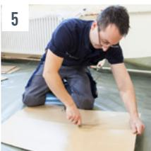
**5** In addition, cut the shortened support panel in half along the broadside. Cut the remaining support plates in half for the first row along the broadside.
