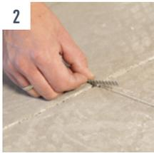
**2** Remove loose edge debris of the screed. Carefully vacuum joints and cracks. Insert the enclosed corrugated links into the cross-cuts.
