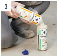
**3** Pour the contents of the component A bottle into the component B bottle and close it. Now mix vigorously for 15 seconds. The consistency can be freely chosen from thin (2 minutes) to highly viscous (6 minutes) depending on the setting time.
