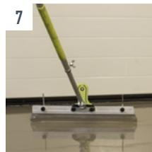
**7** Apply the levelling compound UZIN NC 170 Levelstar to the prepared surface. The raking method (notch size R2) can be used as an alternative to levelling. The screed rake from the UZIN product range is recommended for this purpose.
