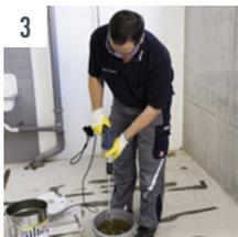
**3** Mix both components with a drill and stirring attachment in the container without streaks. **Now pour this mix into a clean, empty container and mix once more.**
