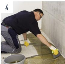
**4** Apply Uzin PE 480 immediately and uniformly with a B2 notch size (min. 500 gm<sup>2</sup>). Now roll over again with the UZIN nylon fibre roller. The UZIN Epoxy Accelerator can be added to UZIN PE 480 to accelerate hardening and thus the continuation of work. Please observe the corresponding product data sheets.
